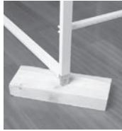
Wood block to protect the floor
